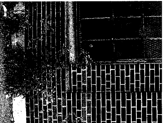
Figure 11 - Dichromatic rug brick, plaster, steel sash window
